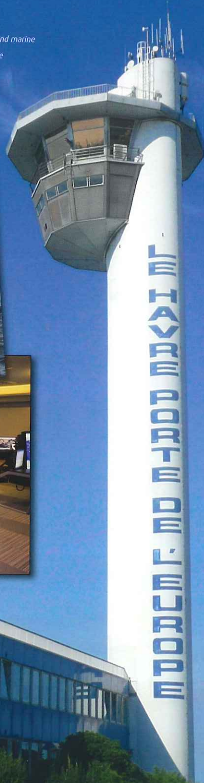
Le Havre VTS Tower.
